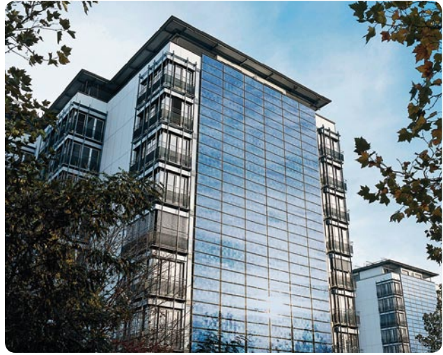
Residential building, 2 x 27 kWp, Freiburg i. Br., Germany
